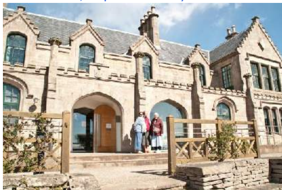
Garrison House, Millport: community hub
