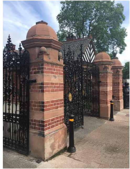
Example of restored gate pillars and metalwork: Botanic Gardens, Glasgow
