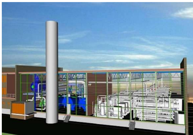
Large district-wide natural heat pump system, providing 13 MW for Drammen, near Oslo, Norway. (Star Refrigeration Glasgow, n.d.)
